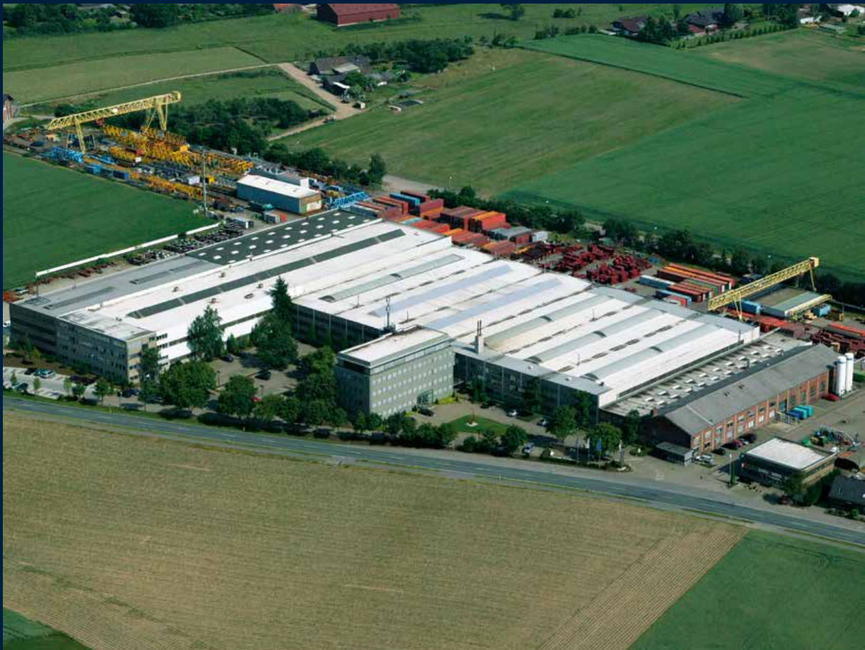
AUMUND Headquarters in Rheinberg, Germany
